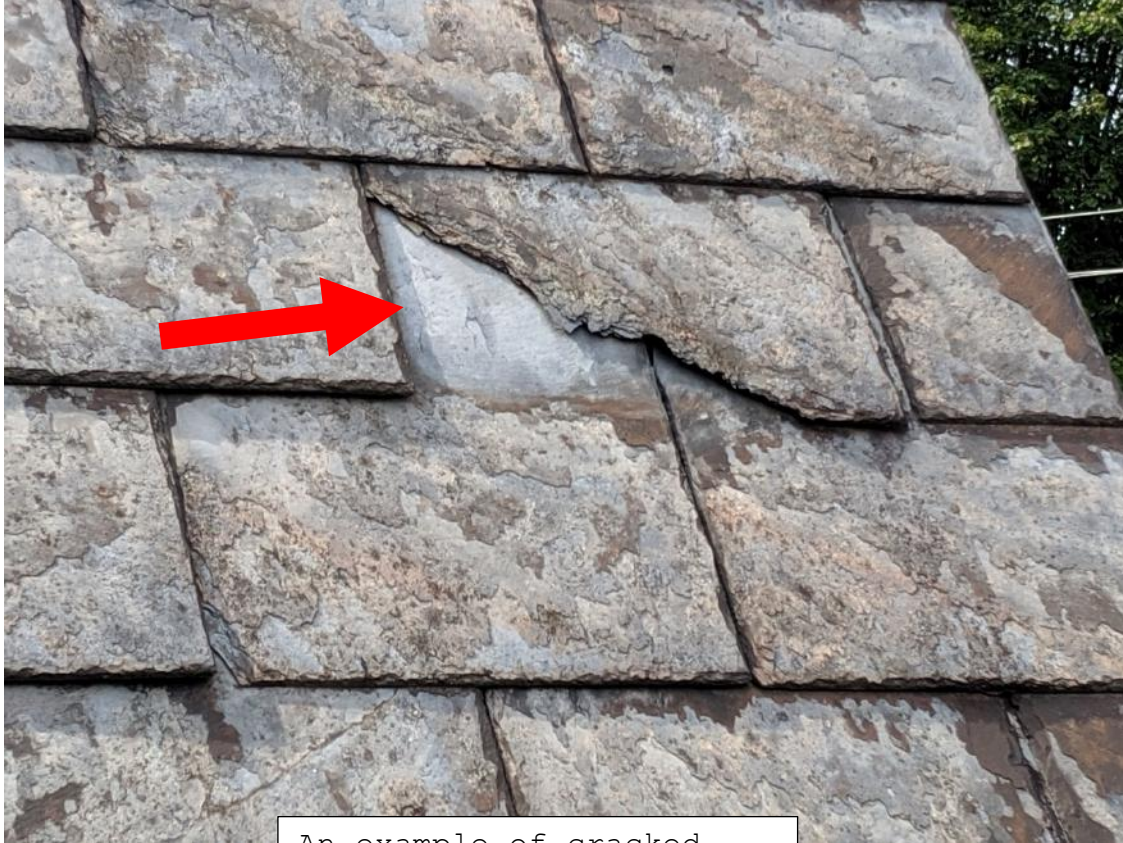
An example of cracked and missing shingles.
