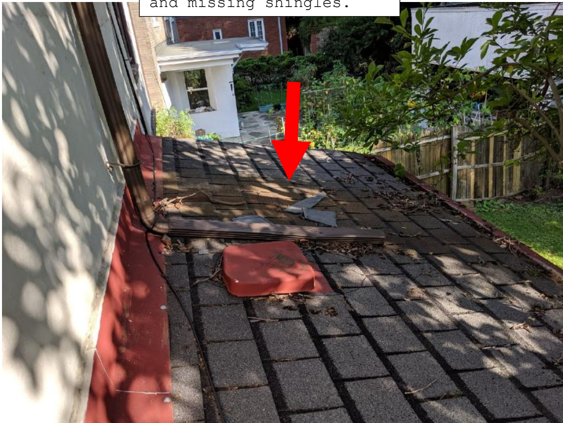
An example of cracked and missing shingles.
