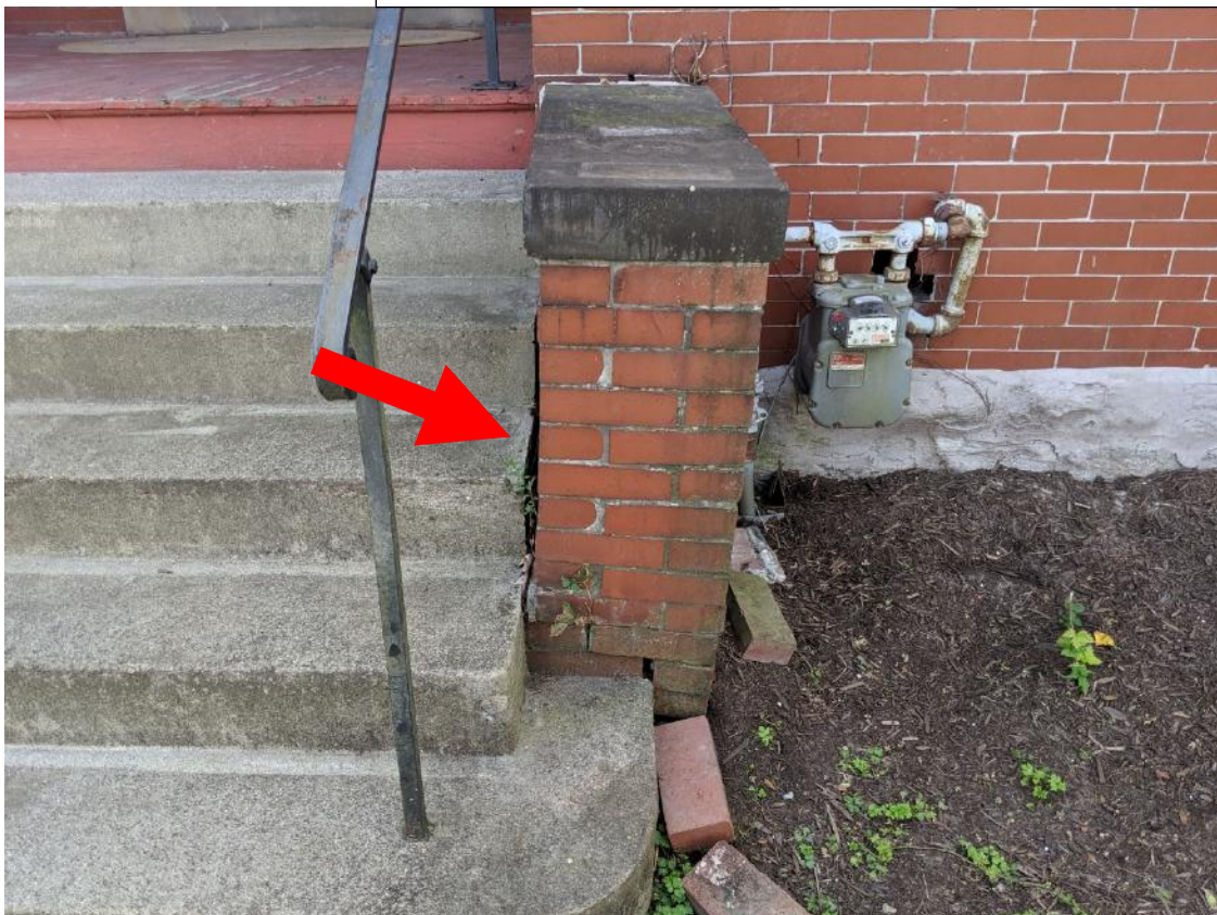
An example of loose brick masonry walls along front porch steps to be rebuilt.
